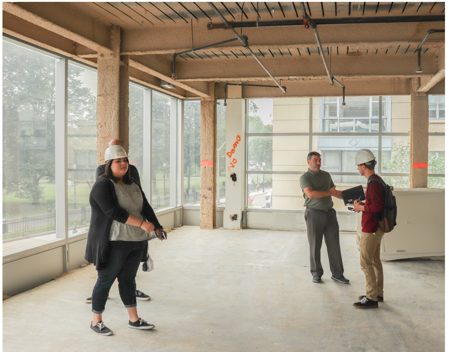
Interior construction on The Commons should begin by the end of the week, pending a hearing with the Boston Zoning Commission. Kyle Bray / Beacon Staff
