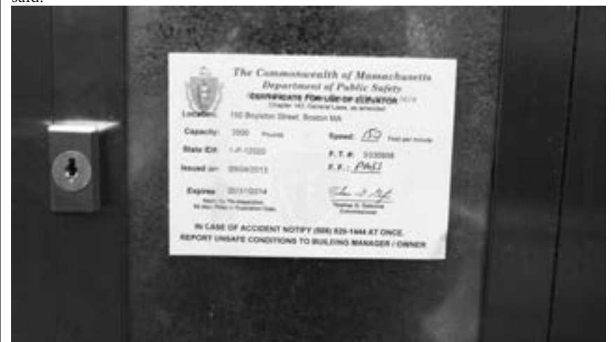
All of the elevators in residence halls passed inspection. • Jackie Tempera/Beacon Staff
